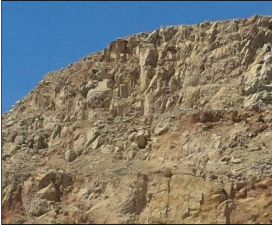
Figure 16-4: Steeply dipping joint sets in the Phase I pit wall that parallel regional fault structures
