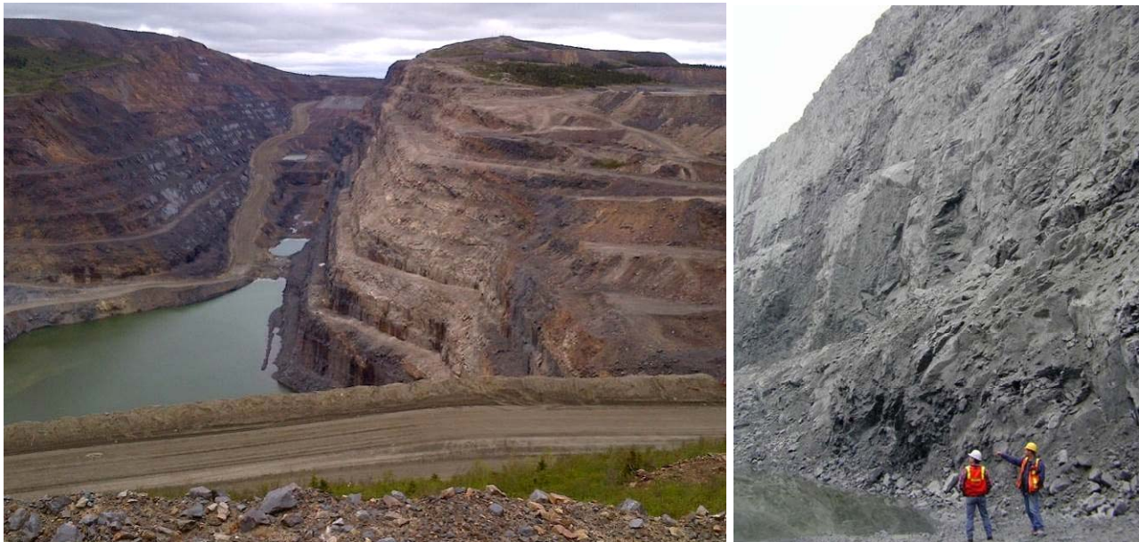
Figure 16-18: Stable pit wall angles achieved with controlled blasting (IOC - Humphrey pit on left 2 , Lac des Iles pit on right)
